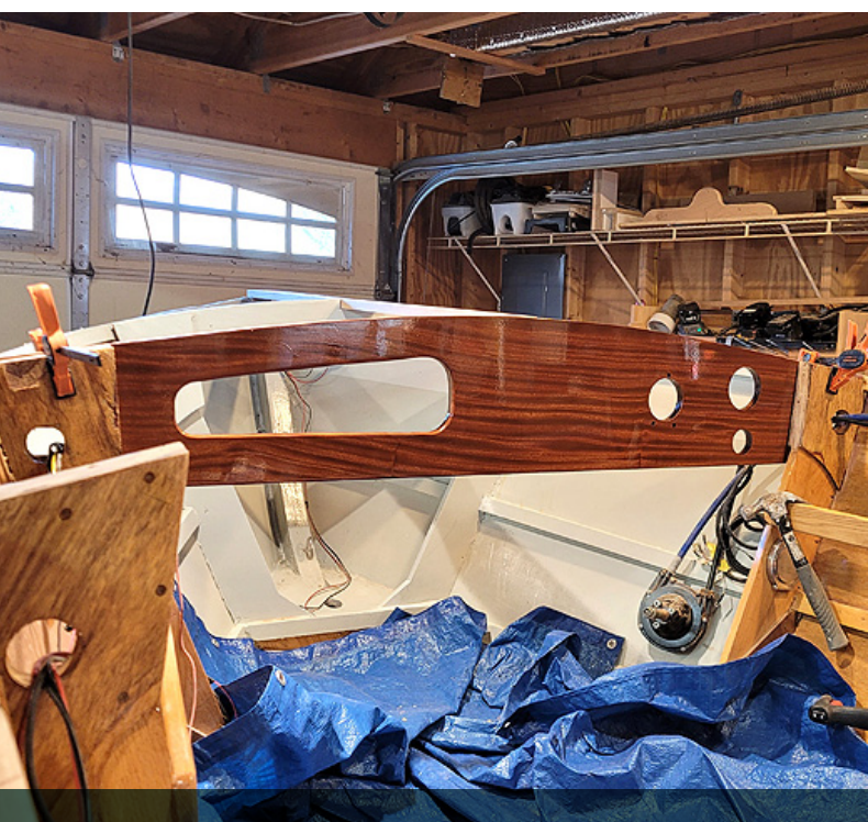
Old deck is removed and the new dashboard is in place
