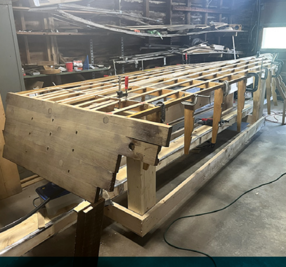
The transom, made from reclaimed teak planks from the Battleship New Jersey, will take its final semi-barrel-back shape once all the battens are in place.
